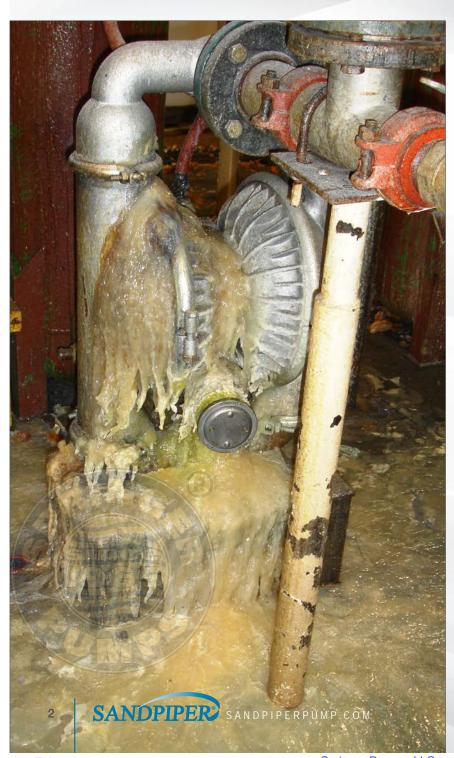
When the pumping diaphragm is breached, the fluid enters the air distribution system and escapes into the environment through the muffler, requiring immediate service.
